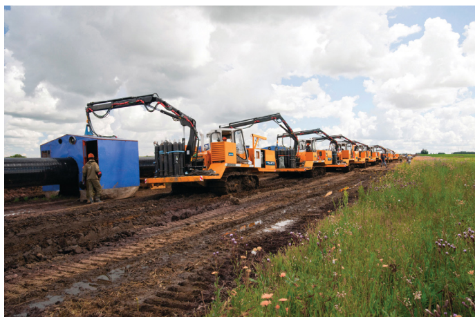
Figure 2. A full, large diameter welding spread.
