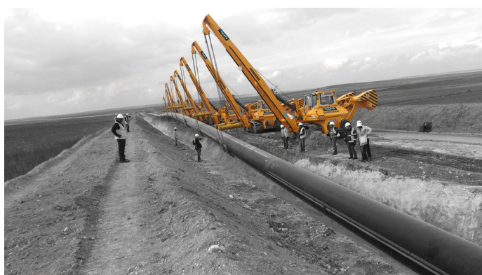
Figure 3. Eight RL64 in action on a 48 in. jobsite in Turkey.
