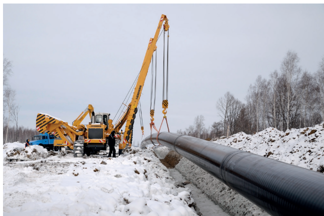
Figure 1. Working in freezing temperatures calls for the right measures. Maats supplies an arctic conversion which allows equipment to work trouble-free in temperatures up to -40°.
